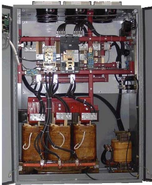
Redundant chargers with common battery compartment
